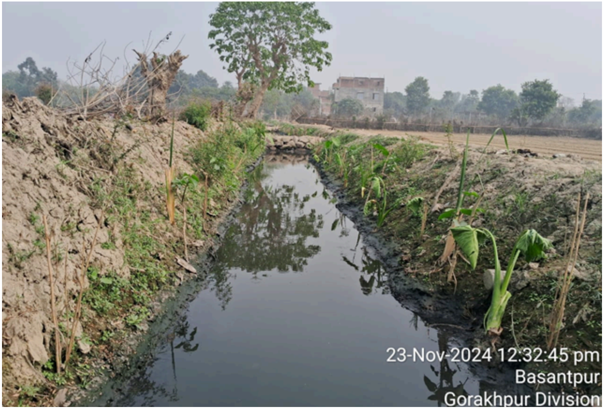
Secondary drain showing rock filters and plants
