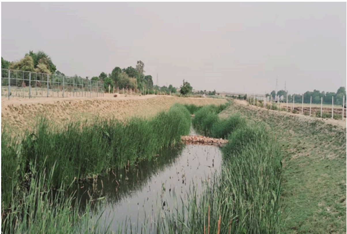
Tertiary drain (Tokia drain) showing aquatic plants between the filters
